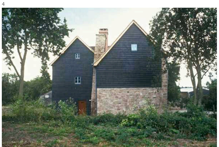
5 Client: The Landmark Trust Contractor: Bevan & Hodges Date: 1983 Value: £800,000
